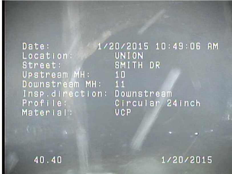
MH10-11_6c5545e6-659f-47fe-9c4d-151a8f7b1ca9_20150120_105632_441.jpg, 00:05:34, 40.40 Manhole, MH11
